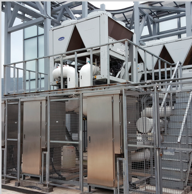
New Air-cooled Chiller Installation with CHW Pumps & Load Bank inside S.S. Enclosure
