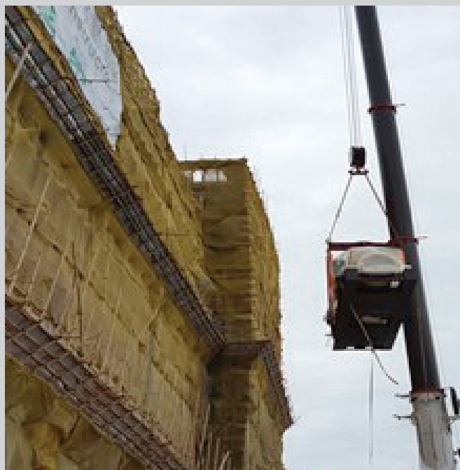
Hoisting Work of Generators and Equipments
