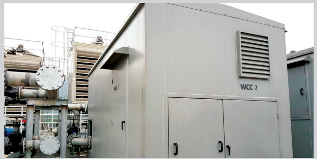
Weather-proof Enclosure for Water-cooled Chiller (TRANE HK)
