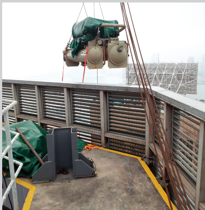
Hoisting Work of Chillers and Equipments
